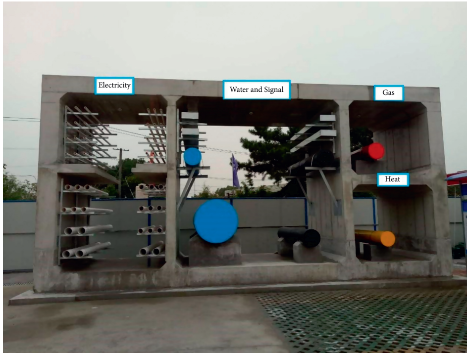
FIGURE 1: Typical section of comprehensive pipe gallery.
