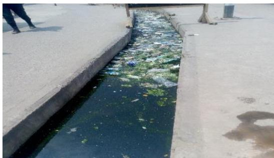
Fig. 5. Total market gutter
