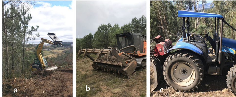
Figure 2. Excavator with a shredder head (a), forest shredder (b), tractor with a crushing implement (c).
