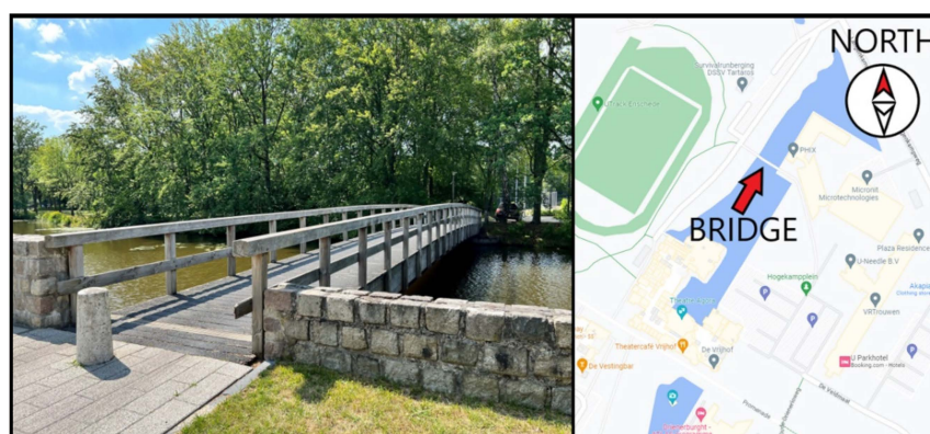
Figure 3. The UT Campus bridge from the east side of Hogekamp (left) and its geolocation (right).
