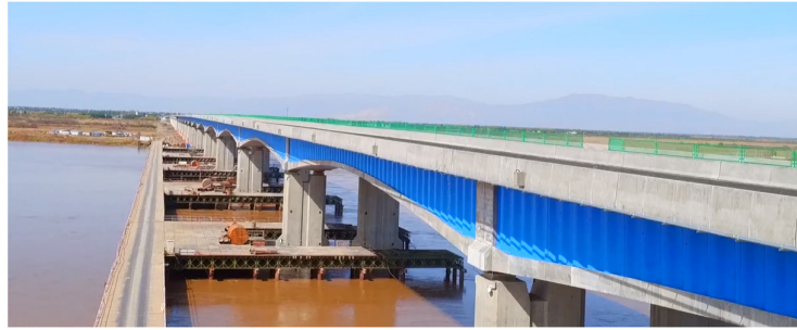
Figure 1. Ningxia Shizuishan Hongyazi Yellow River Bridge.
