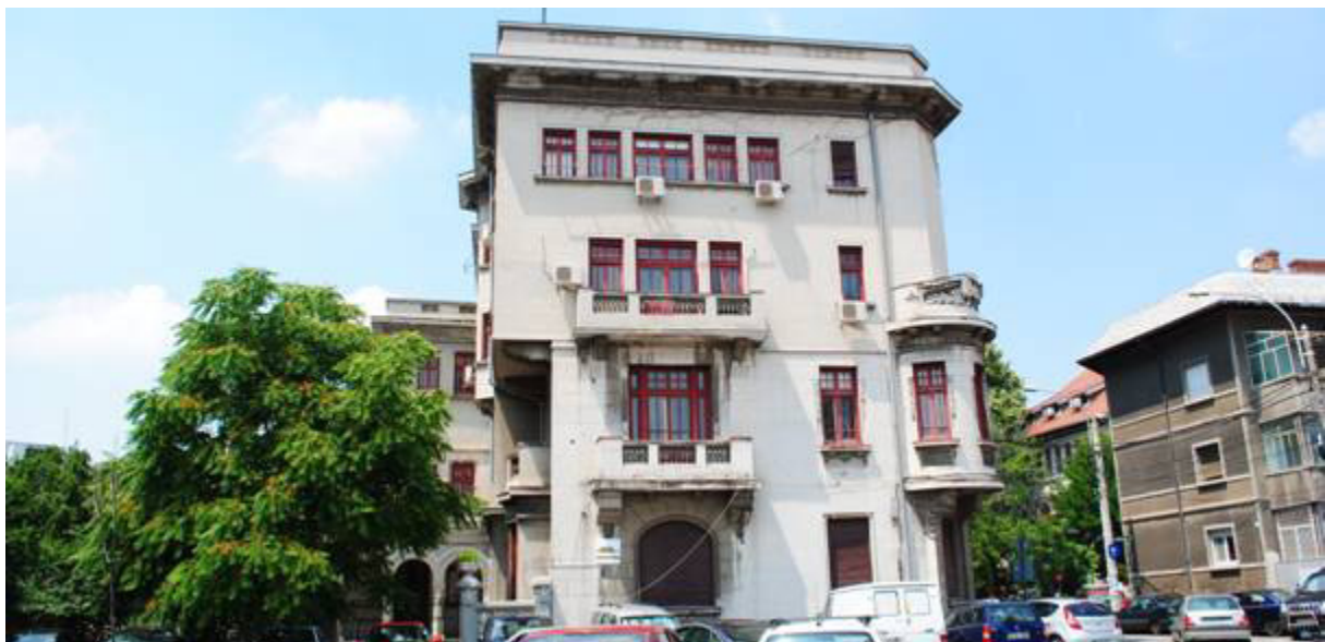
Figure 6. House Rosetti-Solesti, str. Povernei, extension (1928). Photo: M. Bostenaru, 2011
