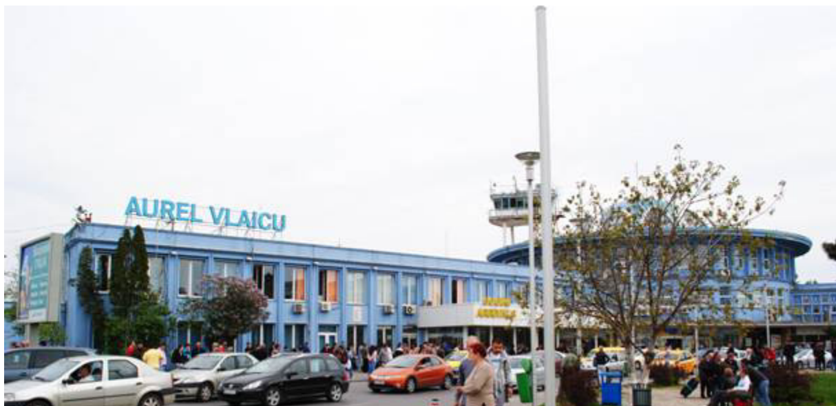
Figure 20. Administrative building Baneasa airport. Photo: M. Bostenaru, 2011
